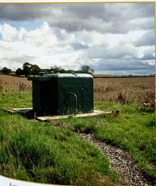
A recently restored nuclear bunker in Yorkshire - a reminder of MAD, Alex Shaw
